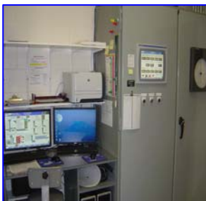
New SCADA (Supervisory Control and Data Acquisition) and PLC (Programmable Logic Controller). This system monitors interprets data and makes changes with all components (flow meter, valve controls, pumps etc.) in the plant and distribution system, it monitors and controls the treatment process. It also collects, stores & trends information.
