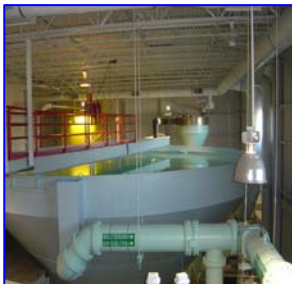
The main influent line is all new, flow meter, pressure reducing valve & control valve. The line was reduced from a 12 inch to a 10 inch to give us better control.
