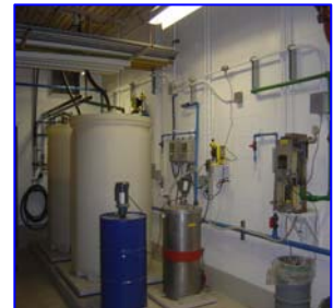
With the plant off line, the chemical feed room was rearranged, with new dual lined chemical storage tanks, new scales which ties into our new SCADA system. An acid resistant floor was applied.
